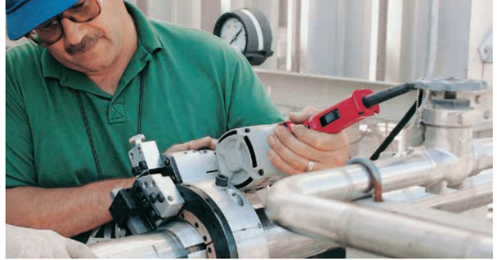
A piping system contractor performing outage maintenance on thin-wall stainless piping system uses an electrically powered SB clamshell fitted with full support pads. The piping system was part of an auxiliary high purity nitrogen supply line at a semiconductor manufacturing facility. A prefabricated pipe assembly was then orbitally welded in place without any additional end-prep being required.
