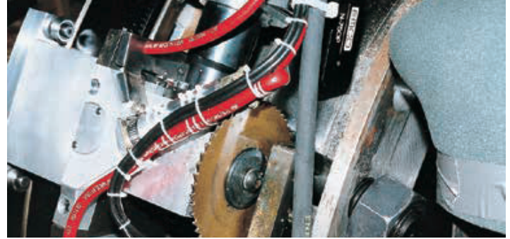
Clamshell mounted saw with video camera, designed for remote seal repair in a nuclear power plant.
