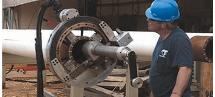
A 600 Series SB Clamshell performing a deep counterbore, critical to a pipe end-matching operation on an Oil and Gas Pipeline project.
