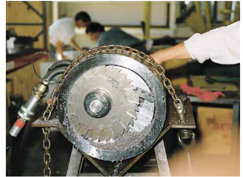
A Tri Tool custom manufactured portable saw with a rotary, eccentric feed that was designed to sever steel pipes that were encased in concrete, from the I.D.
