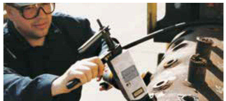
The rugged, ratchet feed, BOILERMASTER steel mandrel and seen rapidly facing torch-cut header stubs.
